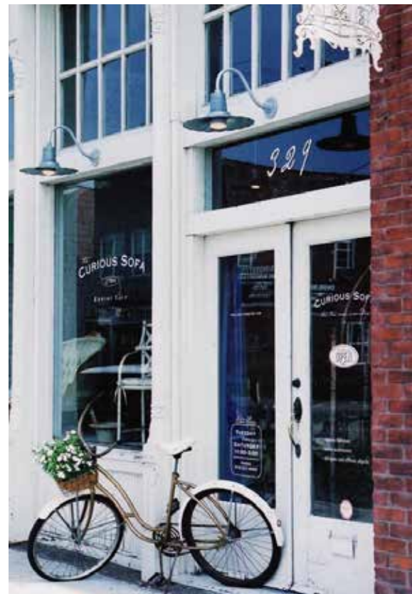
Rehabilitation of historic storefronts and doors.
