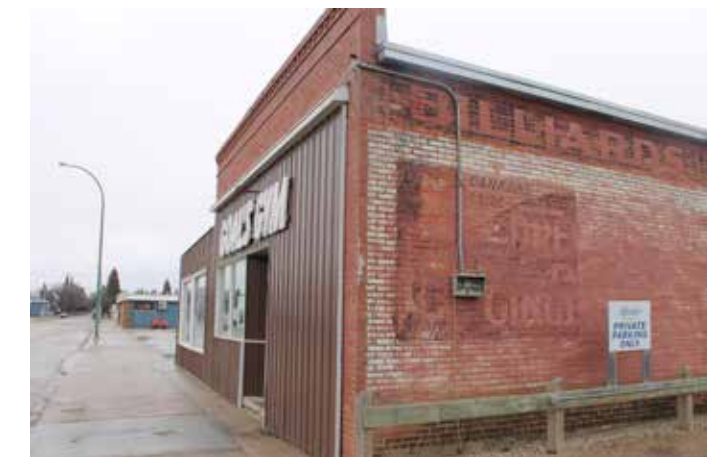
Existing flanking wall "ghost signage" in Melfort.
